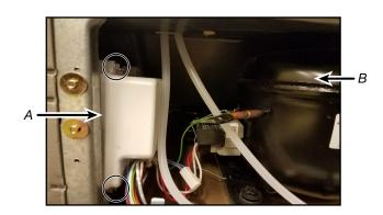
4. To remove the condenser fan, remove the two 1/4" (6.4 mm) hex head screws, disconnect the wiring and lift out.
